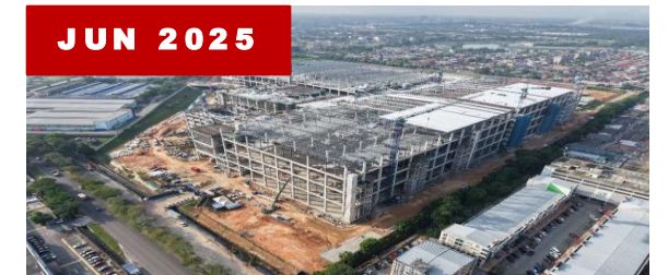
Roofing & envelope works
