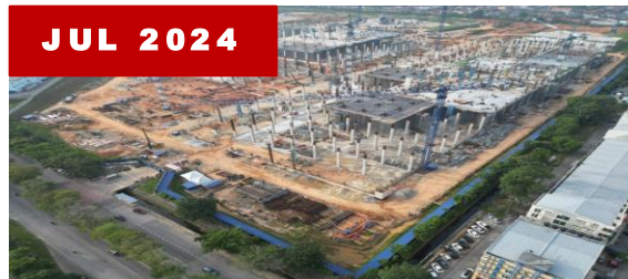
Substructure & column erection
